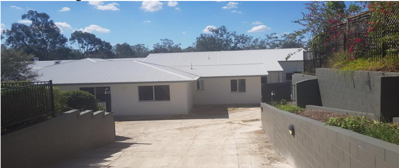
View from driveway
