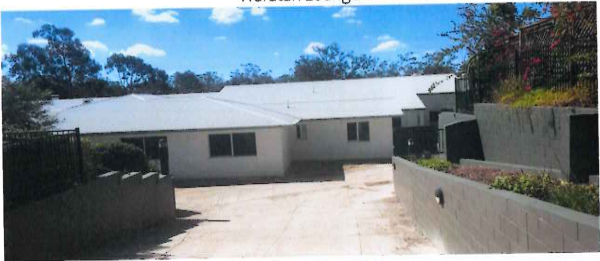
View from driveway
