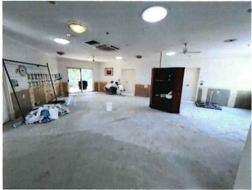
Renovation Progress Lillypilly
