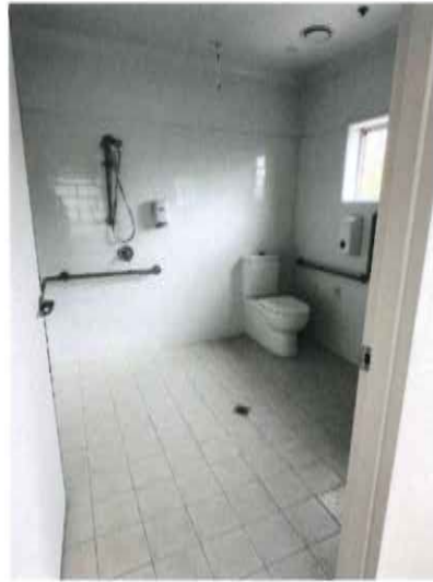
Old Bathroom 76 Now L05 Bathroom November 2024
