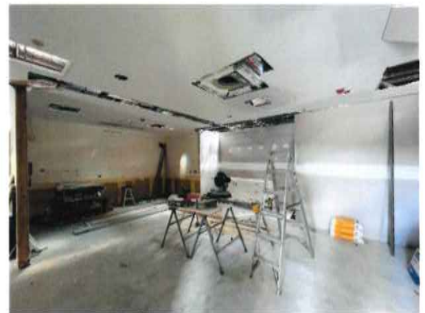
Old Nurse Station & Lounge Room (becoming a dining & lounge room Feb 2025)
