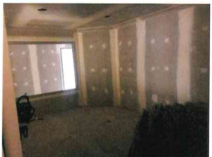
New Waratah Comfort Room
