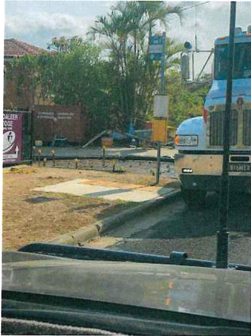
Pouring of concrete driveway
